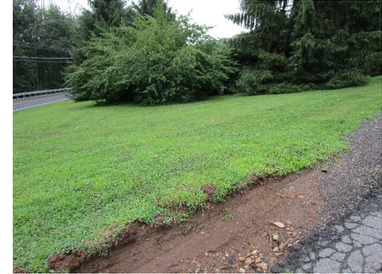
A bioretention system is proposed at the entrance of the property to reduce erosion and infiltrate the stormwater runoff from the parking area. A preliminary soil assessment suggests that the soils have suitable drainage characteristics for green infrastructure.
