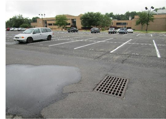
Two mowed detention basins at the east entrance can be retrofitted with rain gardens to capture, treat, and infiltrate stormwater runoff from the driveway and enhance pollinator habitat. Two sections of parking spaces can be converted to porous pavement to capture and infiltrate runoff from the parking lot. A preliminary soil assessment suggests that more soil testing would be required before determining the soil's suitability for green infrastructure.
